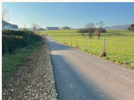
Renewed agricultural road (Rue des Roses /Cité Aline Mayrisch) with an open-pore trench to channel heavy rainfall.
