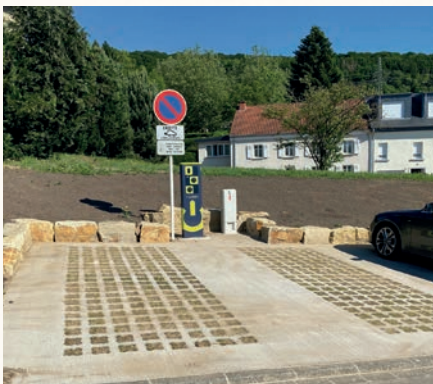
Electric charger "Öko-Cité"
