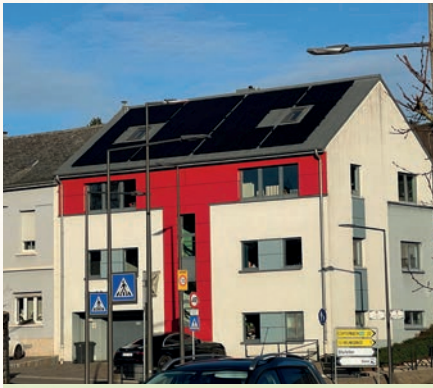
PV installation Scouts Home
