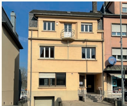
Building (9 rte de Diekirch) for new social services office and commerce
