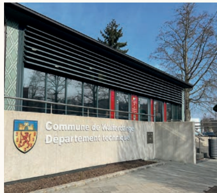
New technical service building
